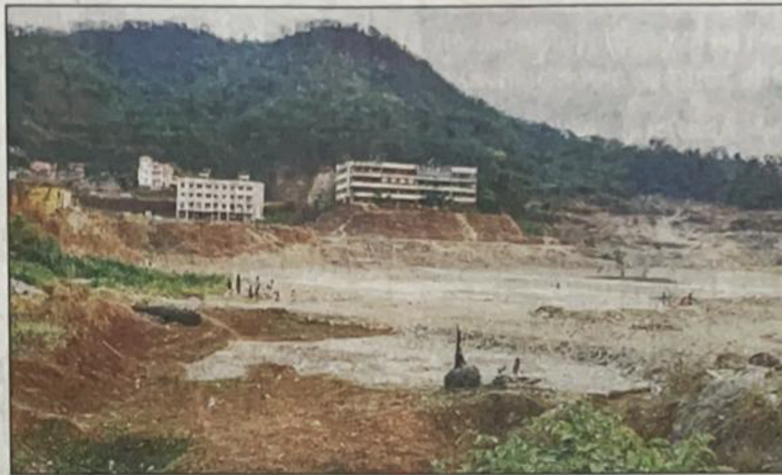
The trust land in Uran's Channe village where excavation work is on
